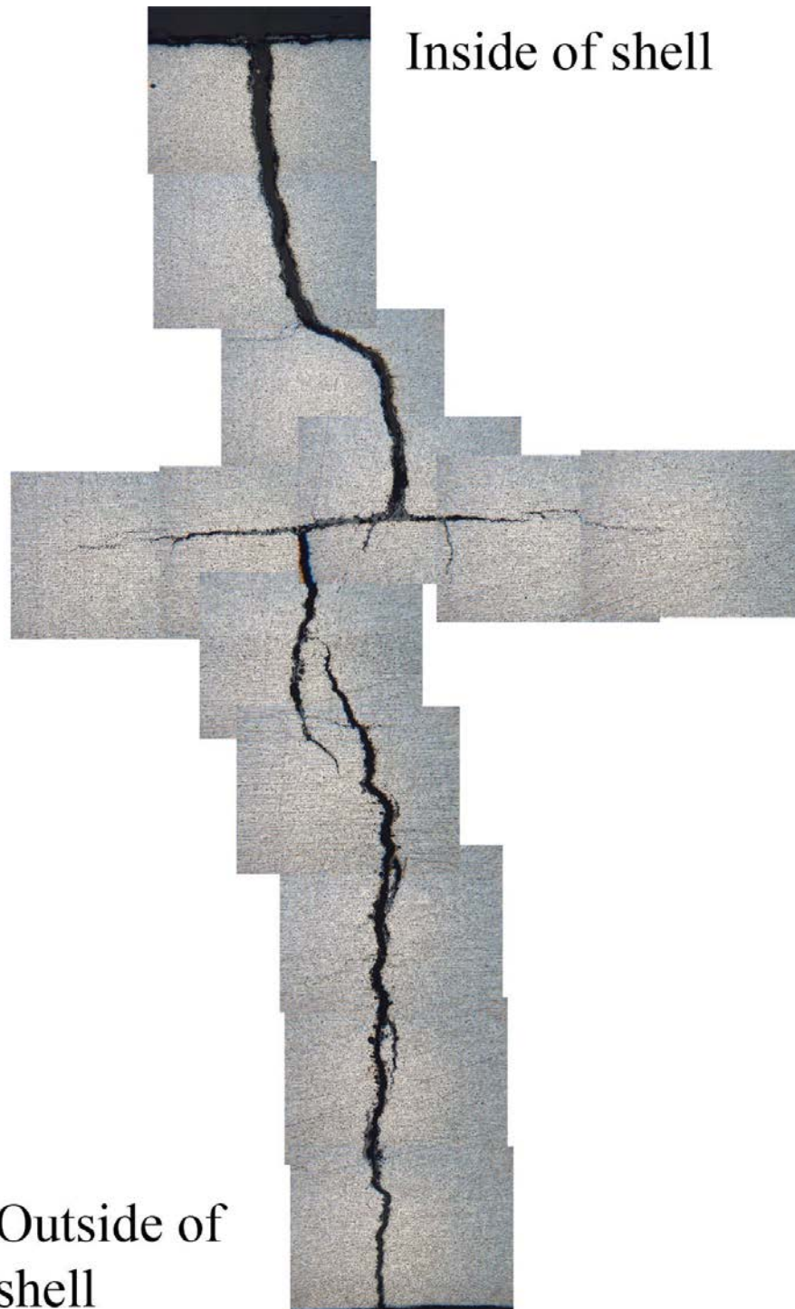
Figure 4 Cracking of the shell occurred from the inside to the outside of the shell. Significant centreline cracking was observed.
